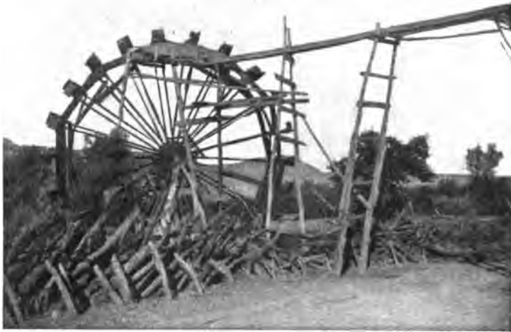
FIG. 113.— WATER-WHEEL FOR LIFTING WATER FOR IRRIGATION, VIRGIN RIVER, SOUTHERN UTAH
